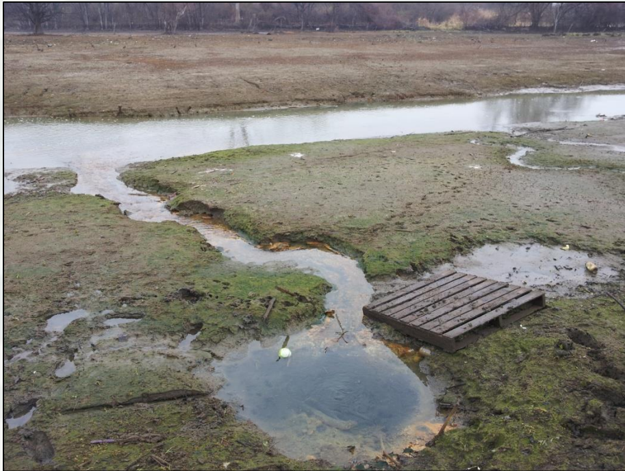
Uncontrolled Underseepage Creating a Sand Boil
