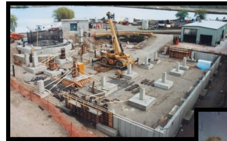
Complex soil conditions
