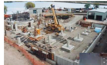
Complex soil conditions
