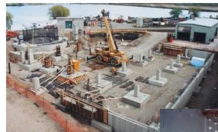
Complex soil conditions
