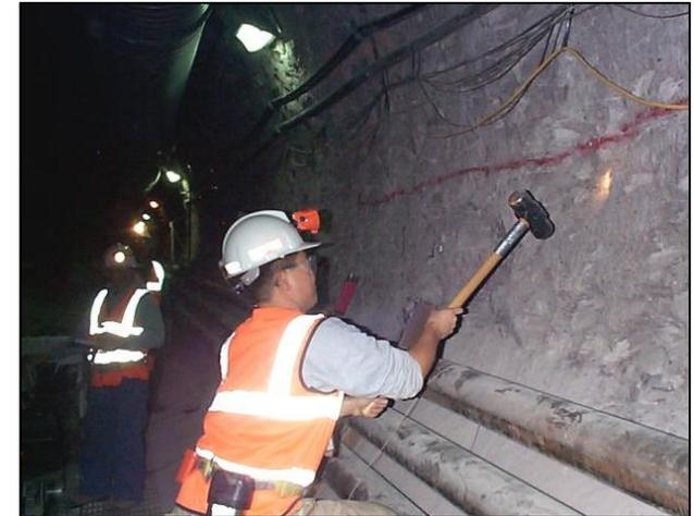
(b) SASW testing within the tunnel
